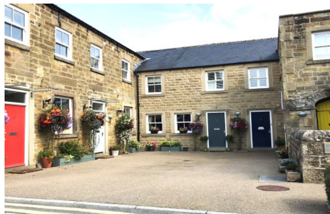
Individual painted doors in courtyard
